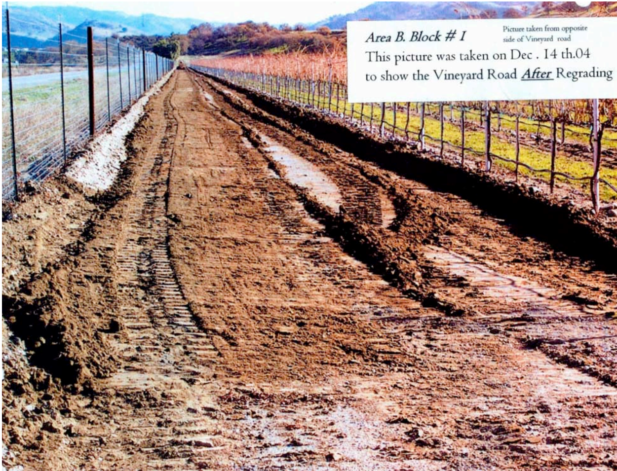
Road at Donati Vineyard after re-grading 12/04
