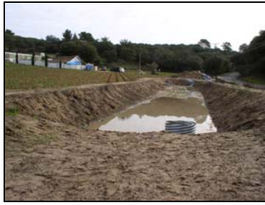
02-004 Before: Roadside drainage and lower field filled with sediment from storm runoff. After: Water and Sediment Basin with straw and grass seed placed on berm constructed in 2003 meters water to roadside ditch and culvert preventing sediment from entering road. The third picture is the rock energy dissipater and overflow for the outlet of the basin into the road.
