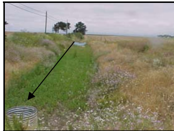
03-003 Before: Sediment from the field and farm roads accumulates next to Highway 1 and continues to flow under the highway through a culvert. After: A Water and Sediment Control Basin continues to slow water runoff and captures sediment before water is released to the culvert under the highway. The third picture shows the outlet riser pipe which meters storm runoff from the basin and the adjacent field.
