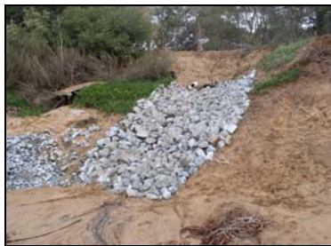
03-002 Before: Makeshift sediment basin installed by farmer. After: New Water and Sediment Control Basin with rock energy dissipater showing the inlet pipe constructed in the upper part of the farm in the fall of 2003. The new basin continues to slow down and capture storm water runoff and sediment from the watershed above the farm.
