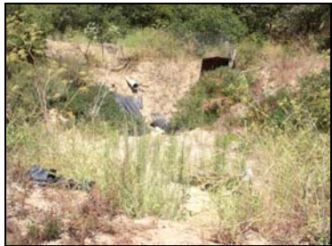
03-002 Before: Makeshift sediment basin installed by farmer. After: New Water and Sediment Control Basin with rock energy dissipater showing the inlet pipe constructed in the upper part of the farm in the fall of 2003. The new basin continues to slow down and capture storm water runoff and sediment from the watershed above the farm.
