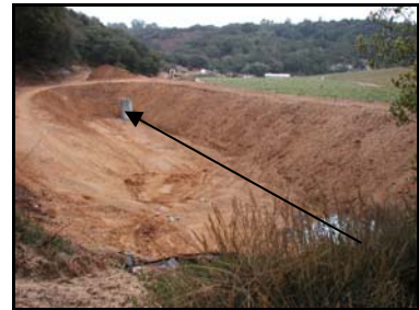
03-002 Before: Makeshift sediment basin installed by farmer. After: New Water and Sediment Control Basin with rock energy dissipater showing the inlet pipe constructed in the upper part of the farm in the fall of 2003. The new basin continues to slow down and capture storm water runoff and sediment from the watershed above the farm.
