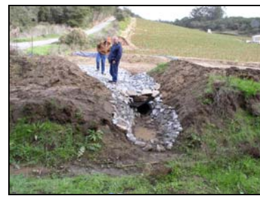
02-004 Before: Roadside drainage and lower field filled with sediment from storm runoff. After: Water and Sediment Basin with straw and grass seed placed on berm constructed in 2003 meters water to roadside ditch and culvert preventing sediment from entering road. The third picture is the rock energy dissipater and overflow for the outlet of the basin into the road.
