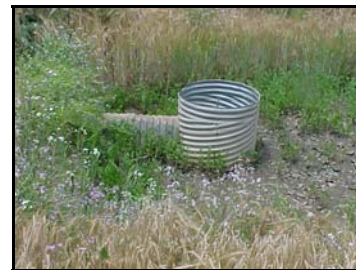
03-003 Before: Sediment from the field and farm roads accumulates next to Highway 1 and continues to flow under the highway through a culvert. After: A Water and Sediment Control Basin continues to slow water runoff and captures sediment before water is released to the culvert under the highway. The third picture shows the outlet riser pipe which meters storm runoff from the basin and the adjacent field.
