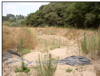
03-005 Before: The first picture shows an existing, poorly constructed Water and Sediment Control Basin. After: Repaired Water and Sediment Control Basin captures and meters runoff during a winter storm. The basin is part of a complete system which protects the farm roads and edges from accelerated erosion.
