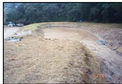
03-005 Before: The first picture shows an existing, poorly constructed Water and Sediment Control Basin. After: Repaired Water and Sediment Control Basin captures and meters runoff during a winter storm. The basin is part of a complete system which protects the farm roads and edges from accelerated erosion.
